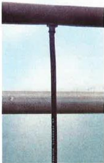
Figure 6. 1/4-inch dropline inserted into spray supply line
